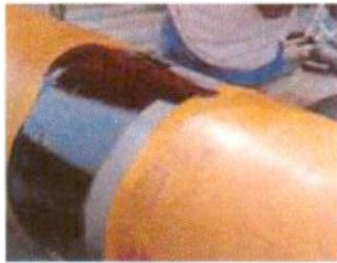
Picture No 5: The Sleeve is then applied over the Joint
