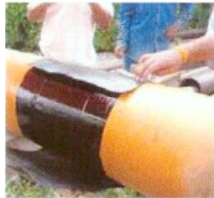
Picture No 5: The Sleeve is then applied over the Joint
