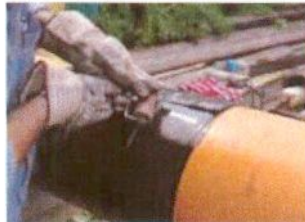
Picture No 6: After shrinking the sleeve , it is rolled to remove air entrapped under the sleeve
