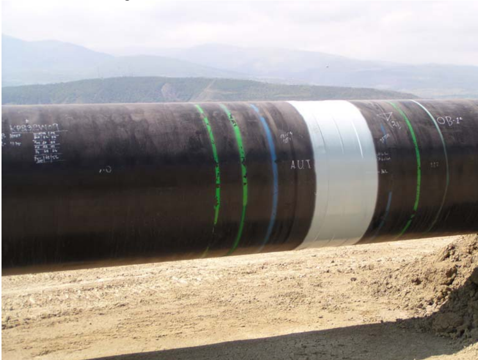
Figure 3. Completed LPE liquid production Girth weld on 3LPE
