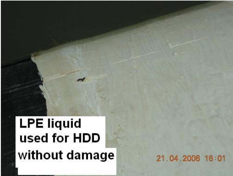
Figure 5B –LPE liquids used on the 3 LPE coated pipes in the HDD BP’s Qandong LNG Dapeng Project China
