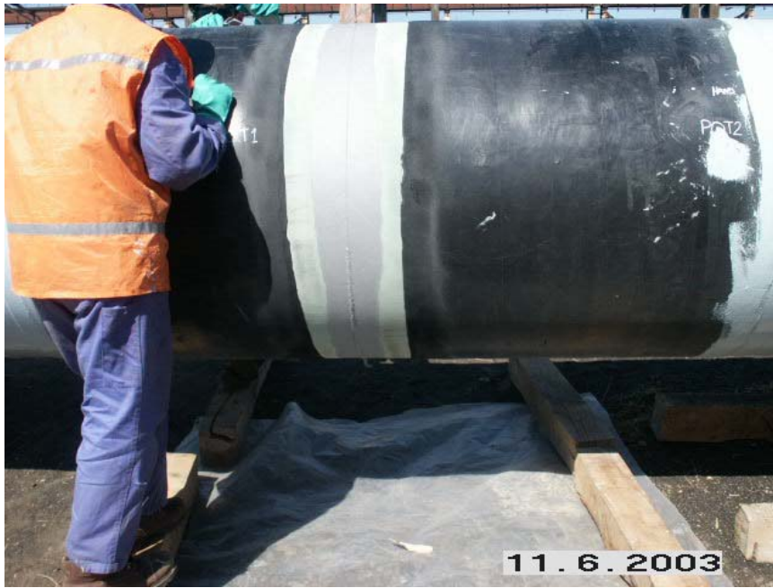
Fig 2 Girth weld with Blasted steel with the FBE Toe
